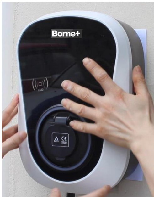
7. Hang the main body of the charging station on the mounting
