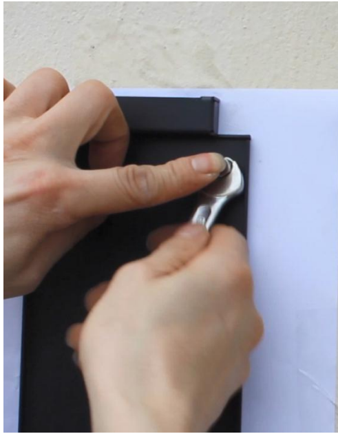
5. Tighten the top screws with a wrench.
